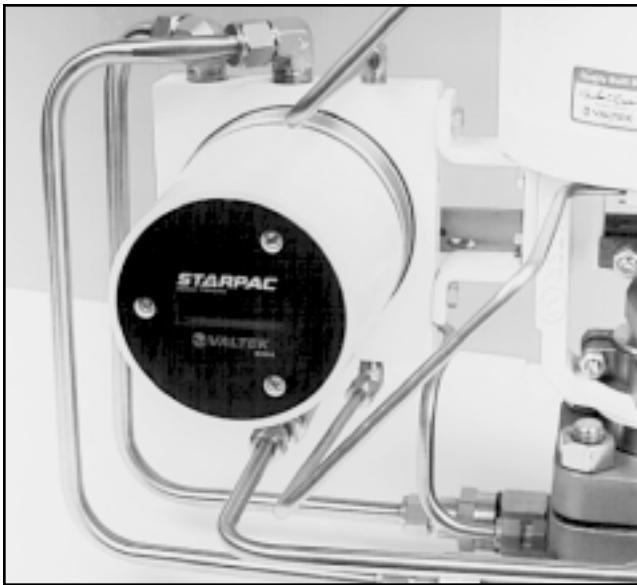
Figure 9: Shroud Retaining Screws / Local Display
