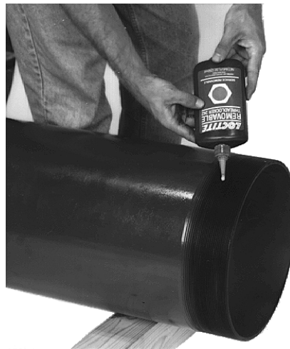
Figure 14 Applying thread locking fluid
