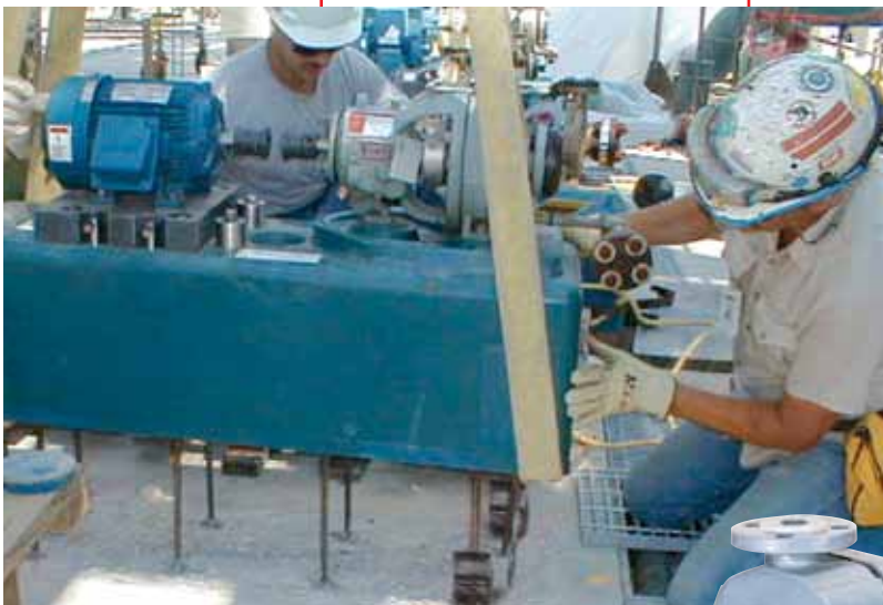
Polyshield installation at a Louisiana chemical plant
