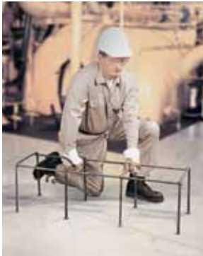
Install rebar cage.
