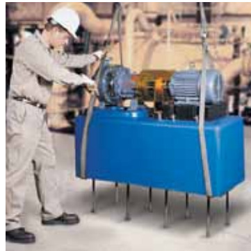
Lower Polyshield over rebar cage.
